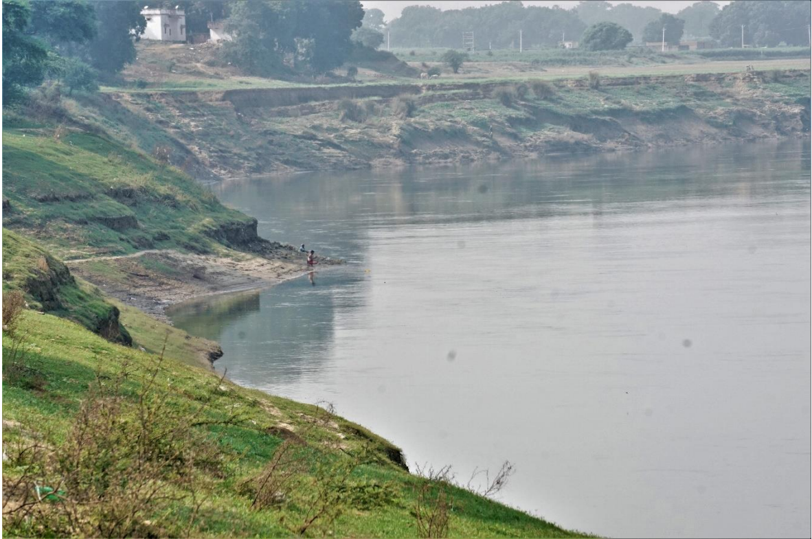
Image 64 : Eroded Bank Near Gaura Khas Village [Right Bank]
