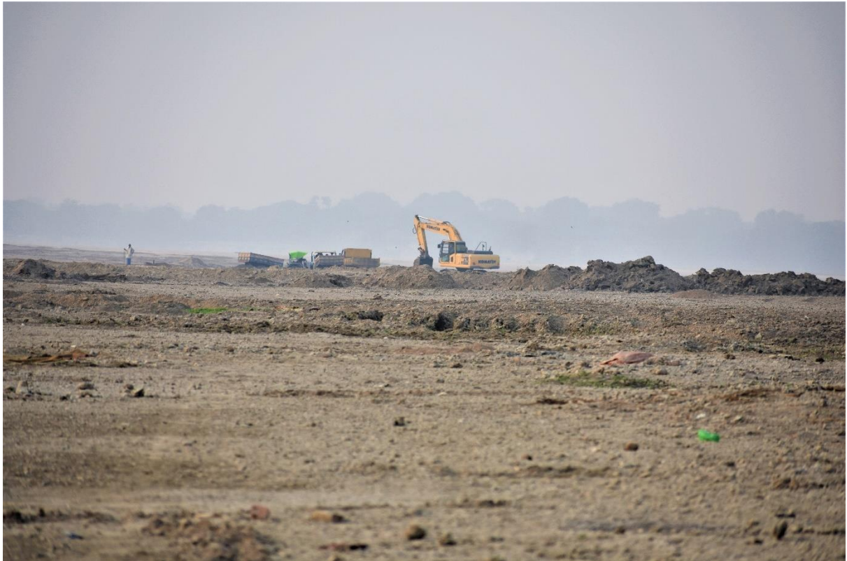
Image 68 : Sand Mining In River Ganga Near Khaira Village
